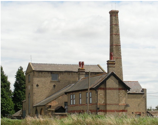
Stetham Old Steam Engine Water Pump 1831
