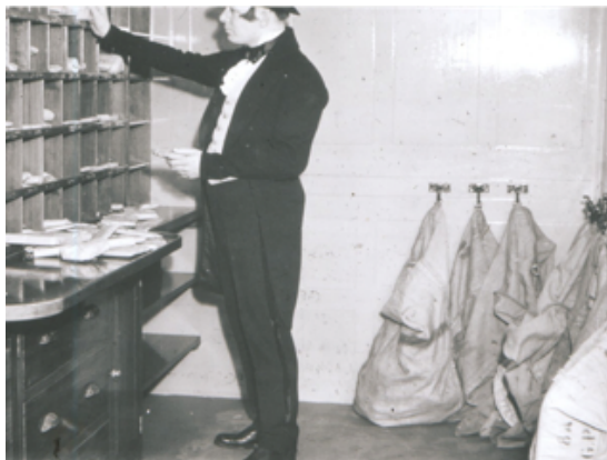
Interior of 1838 TPO replica
