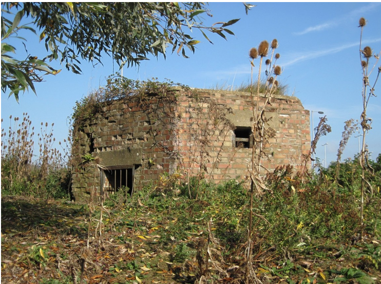
A pill box is still in place at the St Ives park and ride bus station
