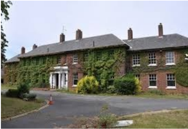
RAF Westwood Officers' Mess before its refurbishment
