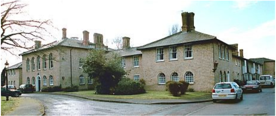
St Ives workhouse as it is today, the exterior much as during its working life
