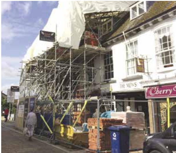
Scaffolding at The Manor House, Bridge Street - David Stewart
