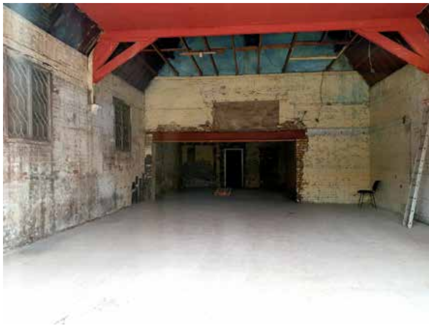
Eastern School Hall showing last two sets of windows, bricked externally.
