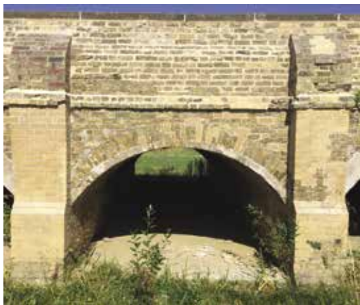
Repaired Archway, the New Bridges - David Stewart
