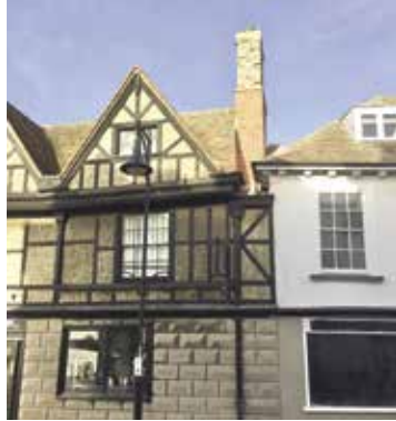
Manor House Chimney - David Stewart
